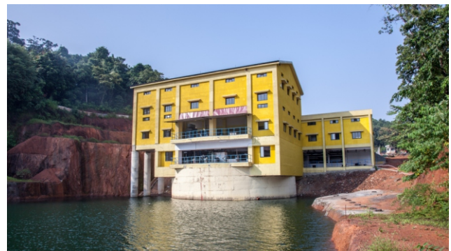
Raw water intake
