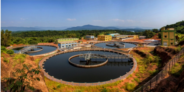
Panoramic view of WTP at Salaulim
