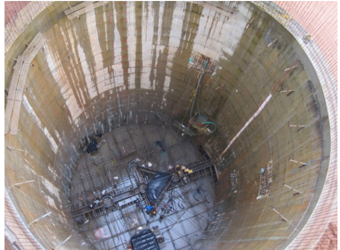
Intake well during sinking operation
