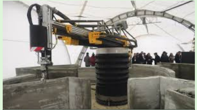
Crane laying down concrete, layer by layer
