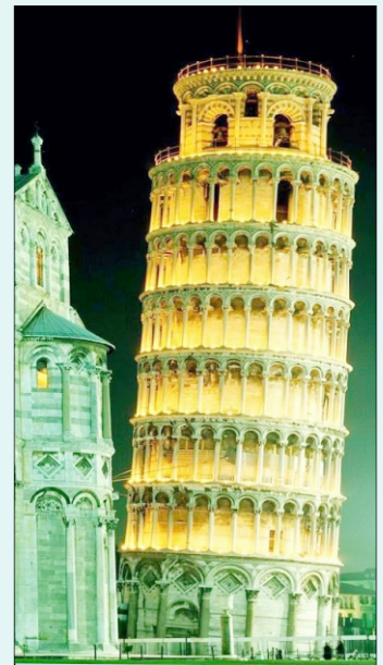
Leaning Tower of Pisa
